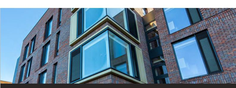
Louvre Guard The Louvre Guard system is a stylish aluminium louvre which can be used with our inward opening SPW300, SPW600 and PURe $^{\circledR}$  window systems. It is ideal for high-rise buildings where excellent ventilation is needed, whilst keeping occupants safe from the risk of falling from a window.
